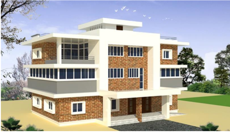
DUDBC MAIN BUILDING, LAMJUNG
